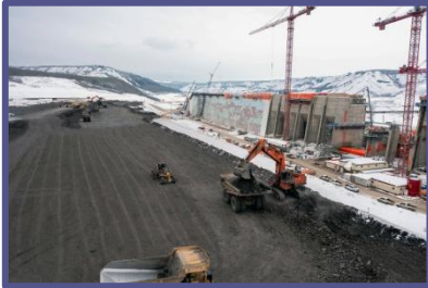
Site C Dam under construction
